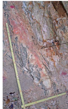
Weathering is advanced along a crevasse
