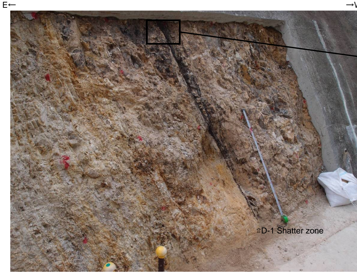
Offscraping of slope (full view) 1m
